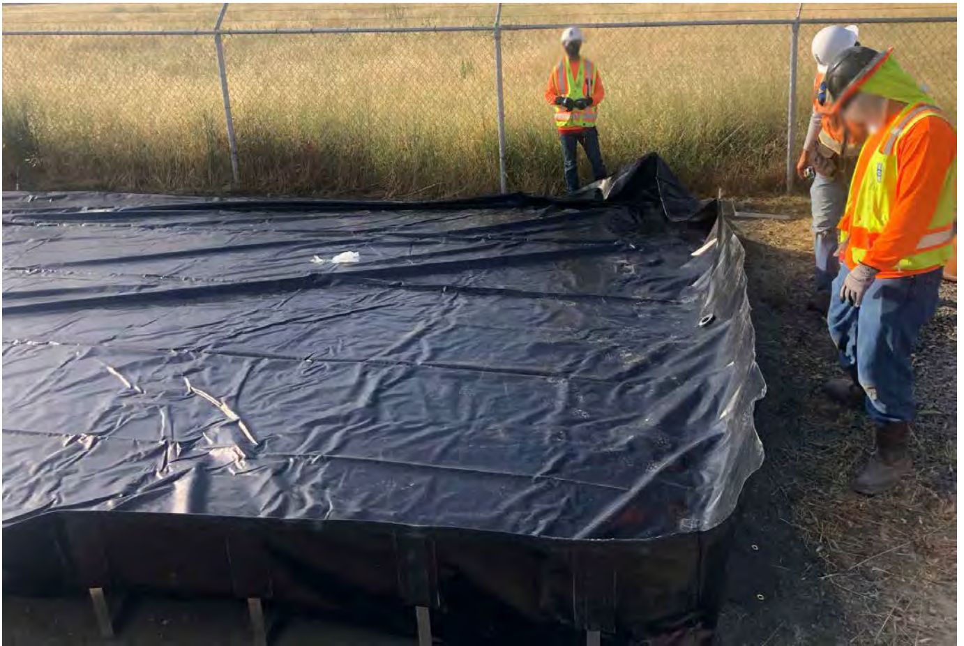
Rolling Out L-Bracket Berm in the Field
