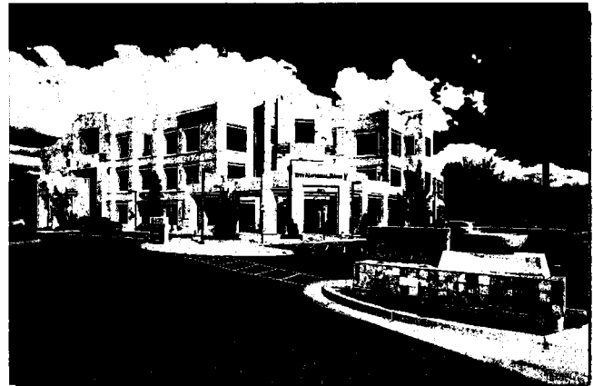
Image 8: Michael Baker's branch office location in South Reno.
