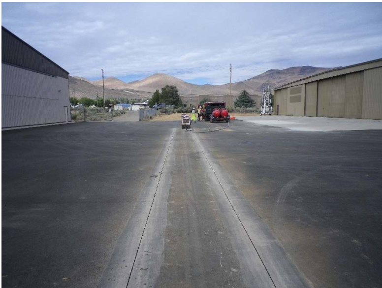
Saw cutting for concrete valley gutter
