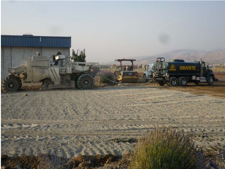
Cement treated base operations
