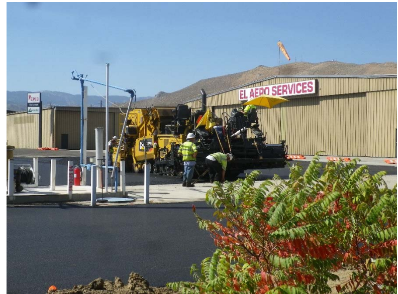
Paving operations near the FBO Fuel facility
