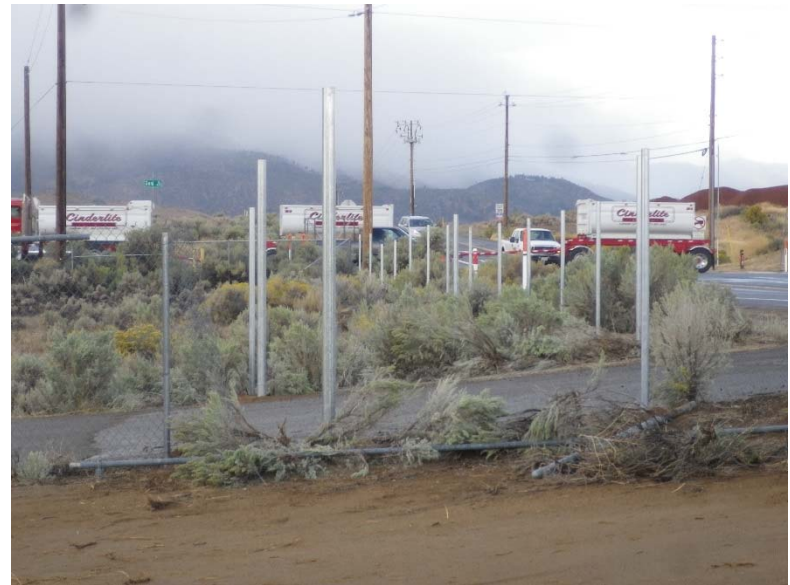
New chain link fence post installed at property line
