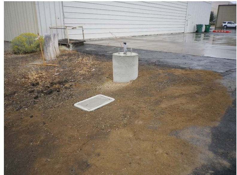
Finished light pole foundation and junction box
