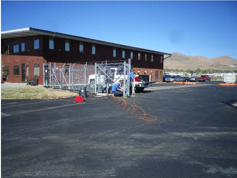
Final touches on the new automatic airport access gate
