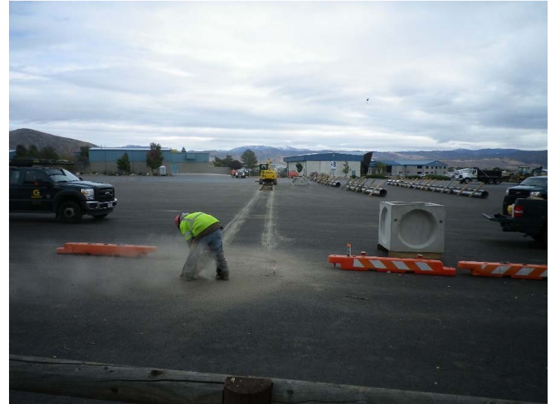
Sawcutting for slotted drain
