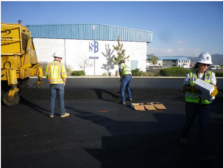
Taking pavement samples for testing
