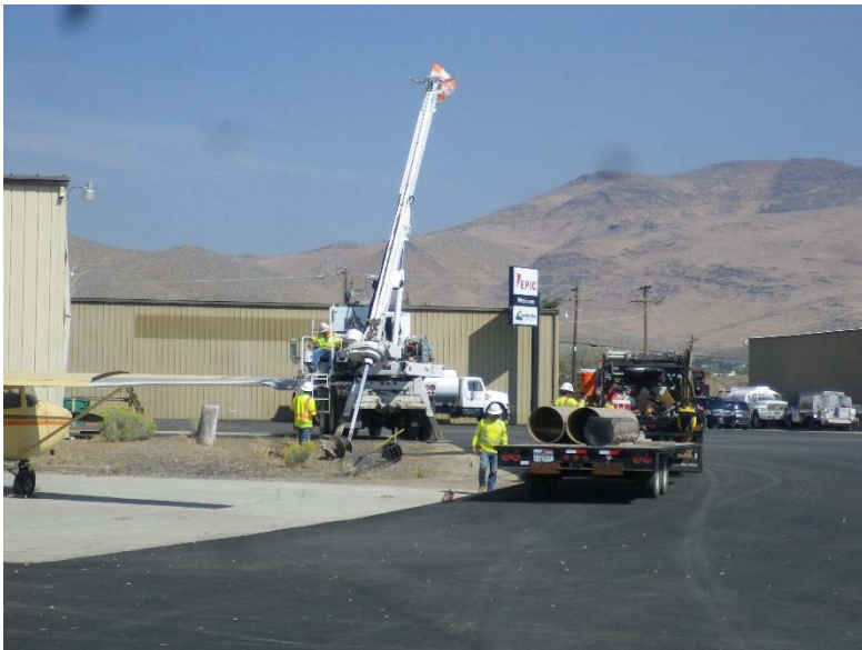
Light pole foundation auger moving into position
