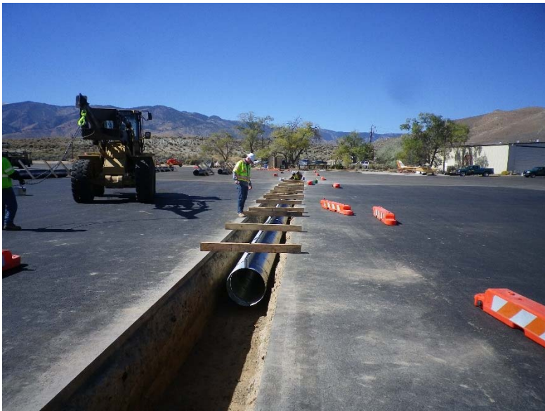
Placing slotted drains
