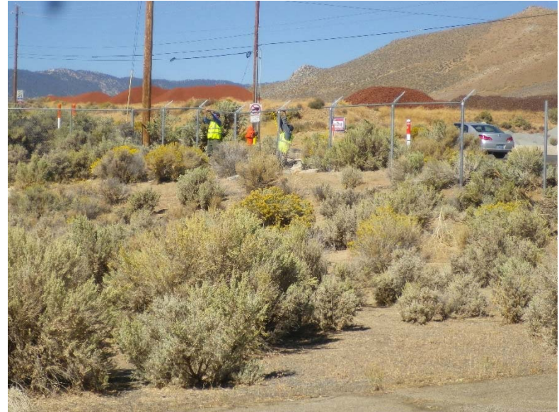
Installing new barb wire on existing fence
