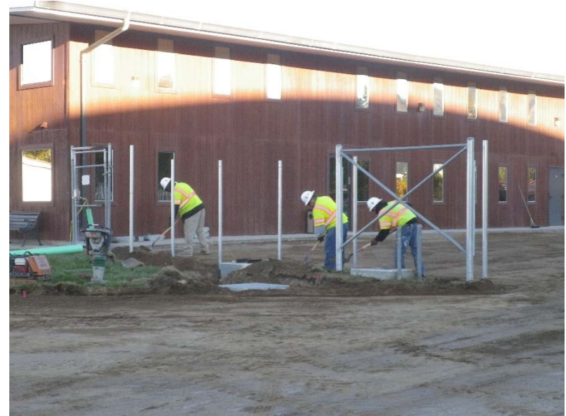
Backfilling around newly installed fence and access gate
