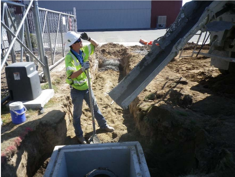
Pouring concrete collar for new drainage feature.
