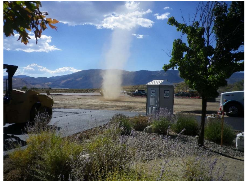
Dust Devil prior to paving operations
