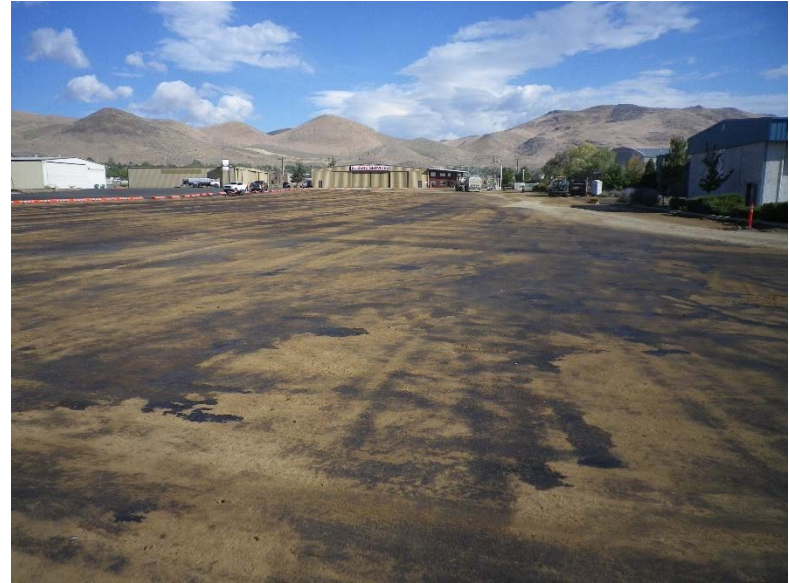
Phase 3 cement treated base curing
