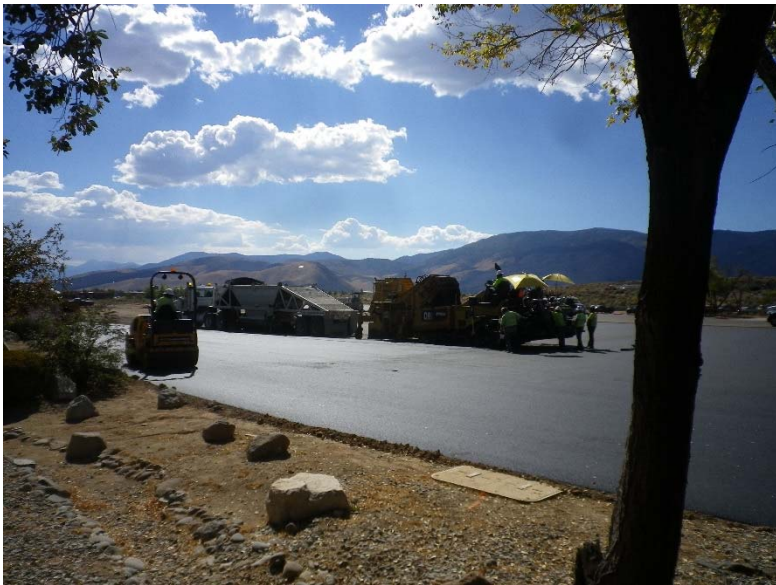
Typical paving operations
