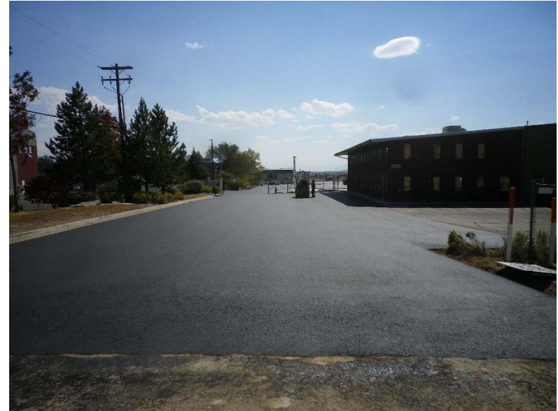
Airport Access Road paved
