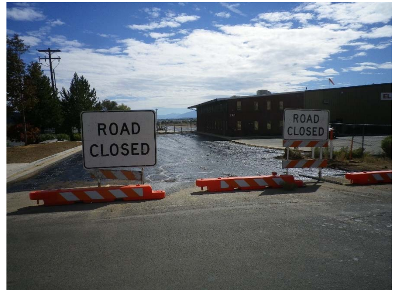
Airport Access Road awaiting pavement
