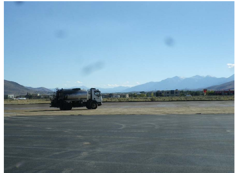
Placing sealant on the newly cement treated Phase 4
