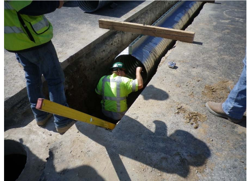
Installing new slotted drain
